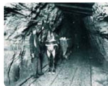
Photograph showing the removal of ore using a horse to pull a train of wagons loaded with salt and potash. Alsace, France. http://www.geowiki.fr/index.php?title=Les_Mines_de_Potasse_d'Alsace_au_fil_du_temps
